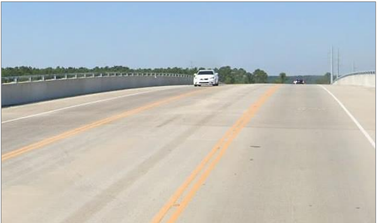
Photograph 16 – Wando River Bridge (facing north)
