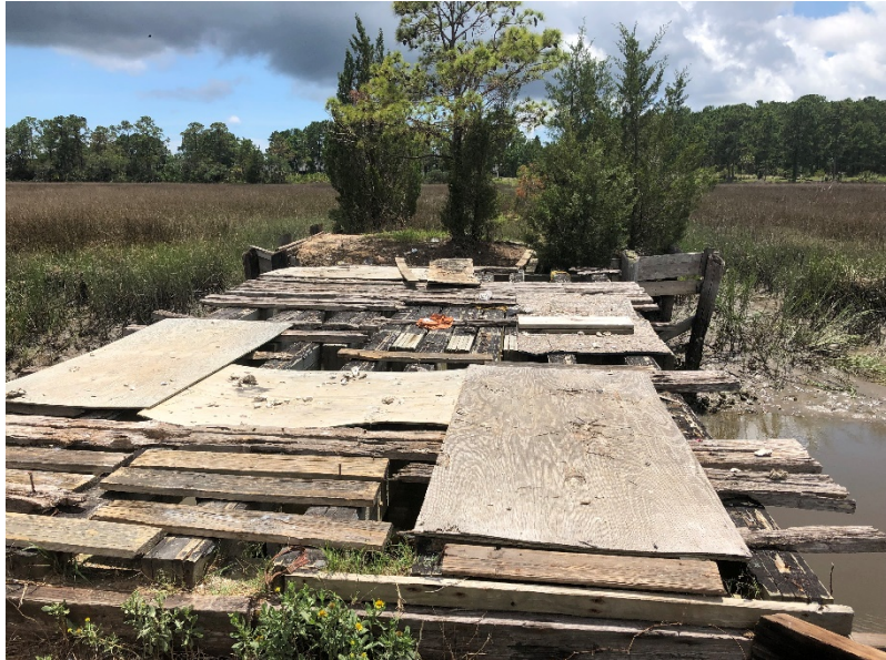
The Bridge over Horlbeck Creek
